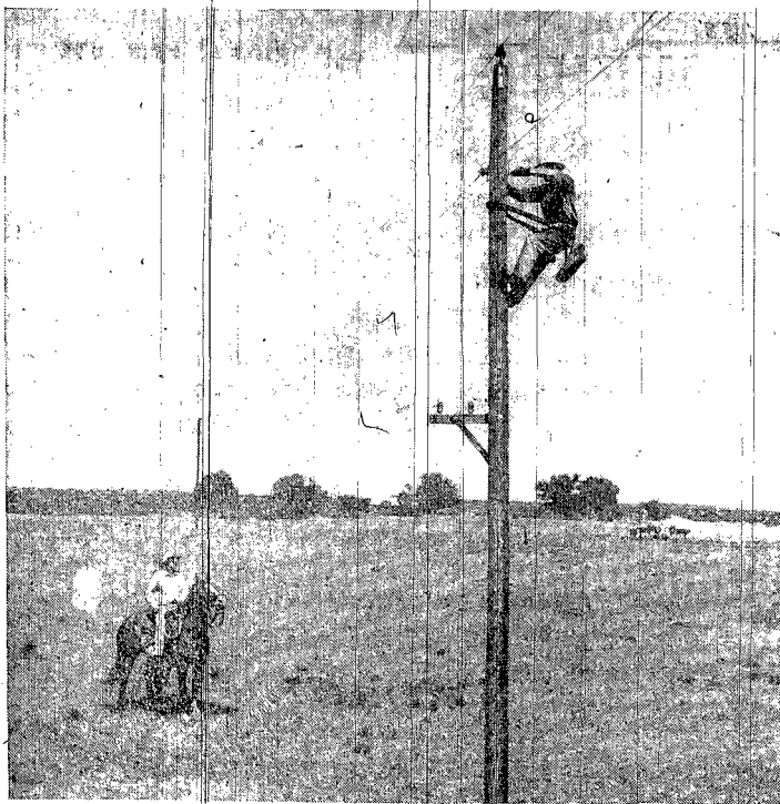
John McGuffin finally gets electricity in 1962, thanks to rural electrification
